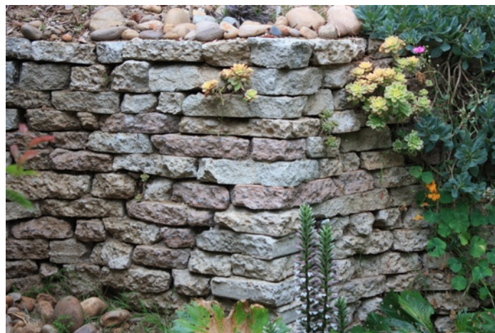
Completed wall incorporating colored concrete pieces
